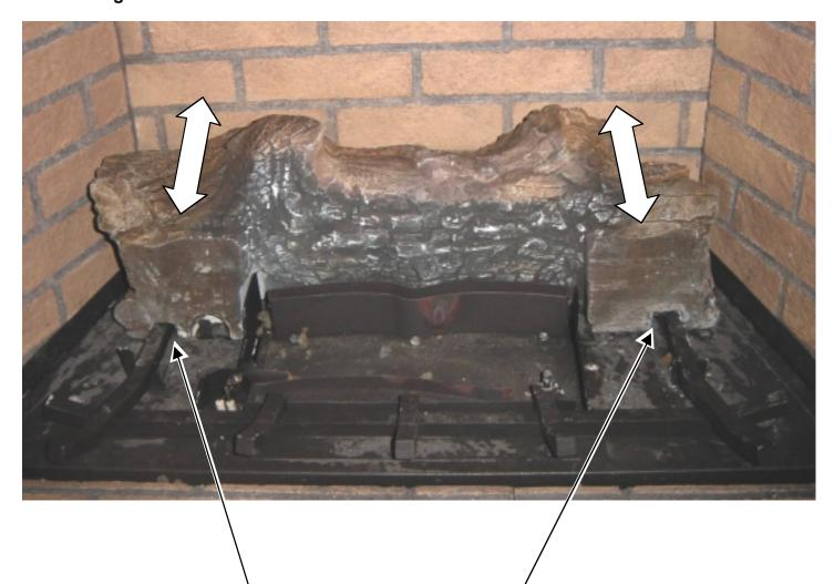
The rear log has two grooves that fit over the grate. These grooves allow for proper adjustment of the rear log. After the logs are in place, and the fireplace has run for 15 minutes, you may wish to verify the log is correctly positioned. You can move the log forward to obtain more glow from the log. If sooting occurs, move the log back.
