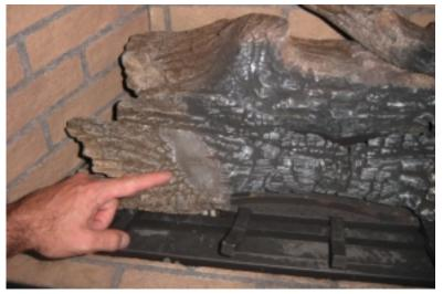
When in place, the log rests level as shown in the picture to the right. Note how the right portion of the log lines up with the right front log, creating the appearance of one log.
