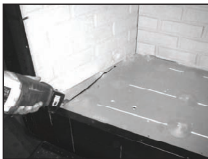
Figure 12.2. Using a sawz-all, cut out the floor.
