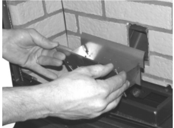
Lift the firepot out of the firebox.
