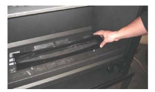
**NOTE**: When replacing the cast burner cover, make sure the notch on the cover fits over the pilot assembly on the right side.
