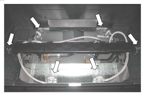
After replacing the accent light bulbs, restore the fireplace to the original configuration. Make sure the burners are correctly positioned and have not been moved (see photo above for reference). When replacing the crushed glass you may want to use a plastic bag to direct the glass around the perimeter of the burner cover (see photo below). The glass should cover the glass tray and be evenly dispersed.
